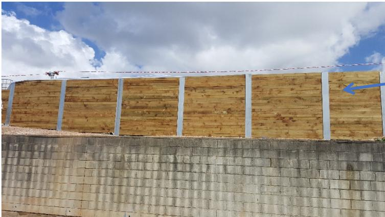
A retaining wall consisting of H columns and timber sleepers was utilised to repair the slope.
